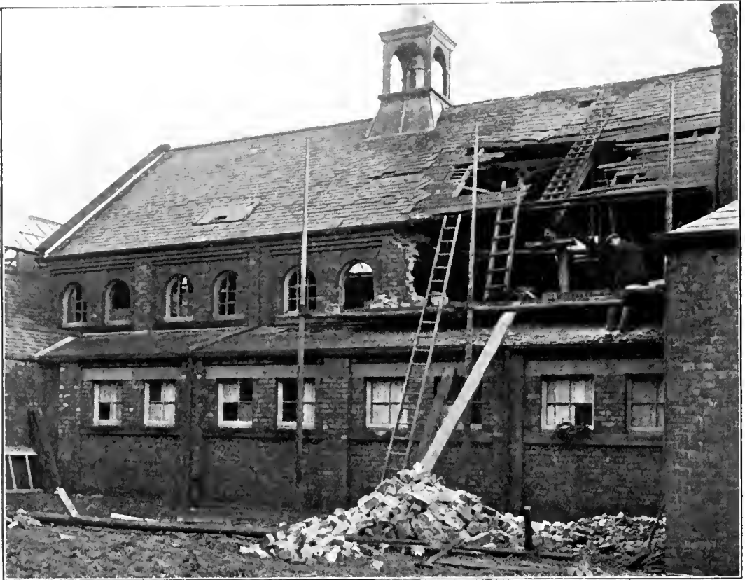
HARTLEPOOL : THE WORKHOUSE DINING HALL. ["Times" Photograph].
